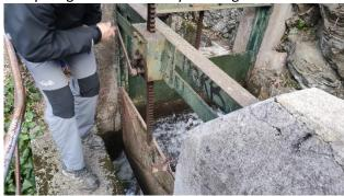
For the distribution of water, every water intake is equipped with a sluice gate that allows control of the flow rate:
